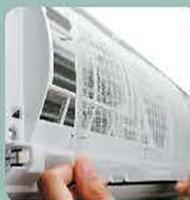
Dust collects on the grille, which is difficult to clean. It also increases the suction resistance, which results in capacity reduction and higher noise level.
